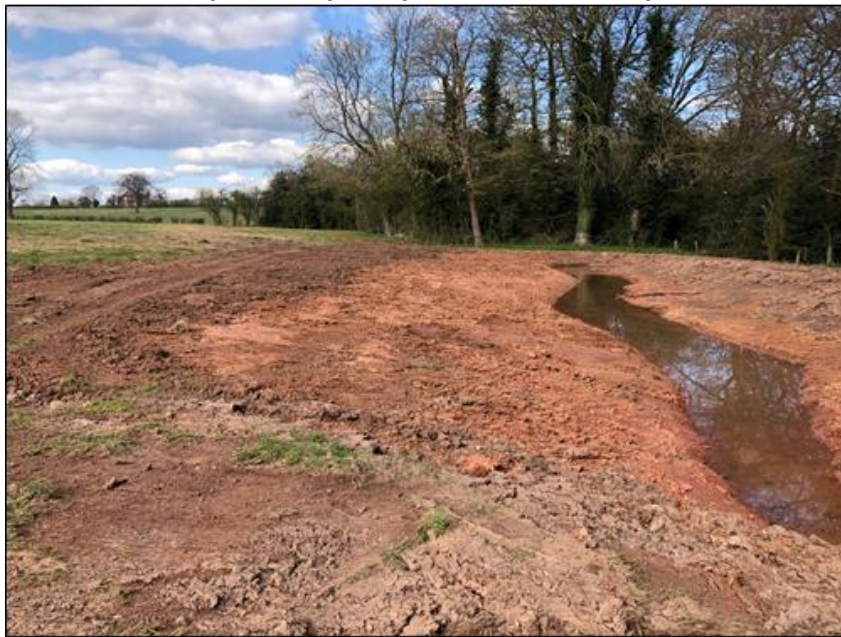
Floodplain scrape, to fill when brook is in flood
