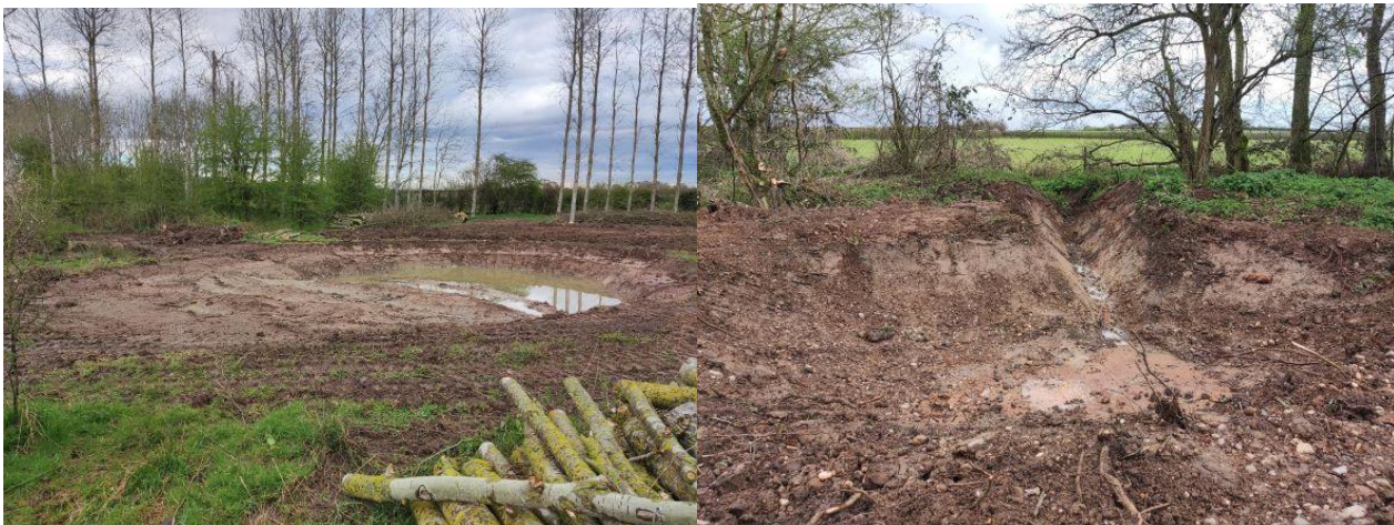
Purlieu Lane backwater pool created 2022
